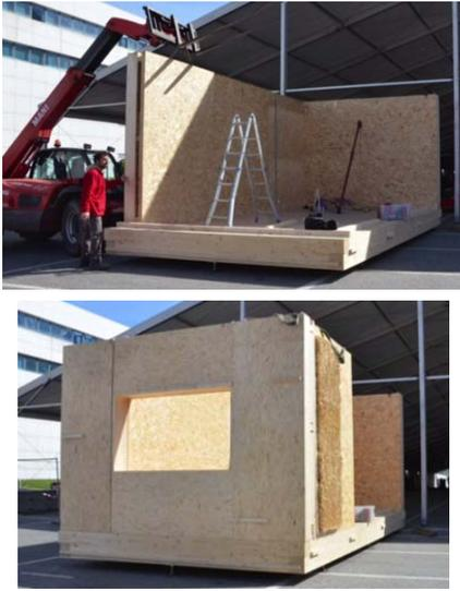
Fig. 1. Housing module assembly.
